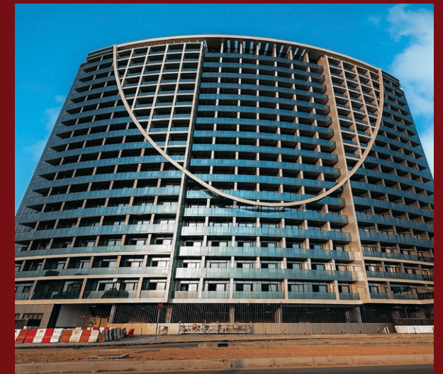
The V Tower
